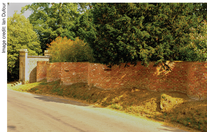
Figure 4: The Bramfield crinkle-crankle or forcing wall
